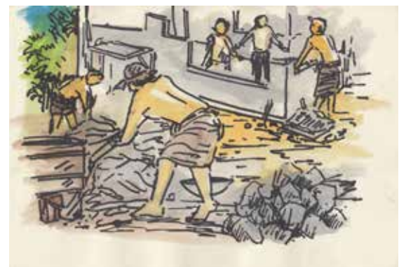
Ajith is constructing the home
